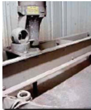
Incoming wastewater is held in the equalization tank, where mixers and air spargers may be used to balance out the solids and minimize BOD formation.
